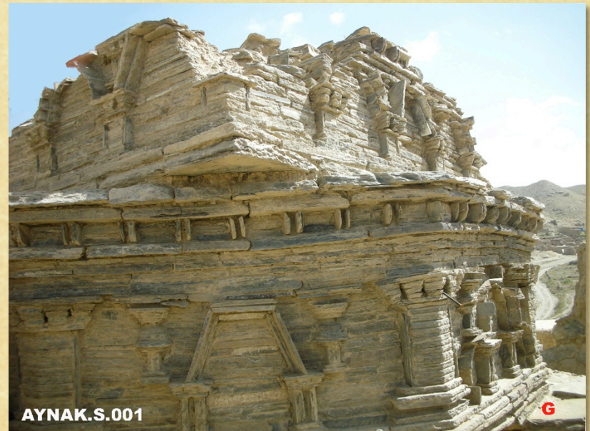
S. 001- Aynak. Kafariah Tapa.: stupa G is a very well built monument with small joined schist slabs and strips.
